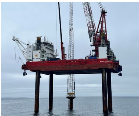
Figure 8. An offshore meteorological mast in Danish waters during decommissioning. Source: Tim Wilms, Vattenfall, presented at SIME 2026.
